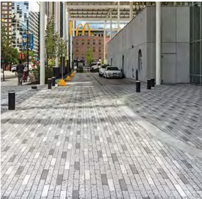
A variety of paving types is proposed (see illustrative plan). Permeable paving would meet the TCC grant requirement for stormwater treatment.
