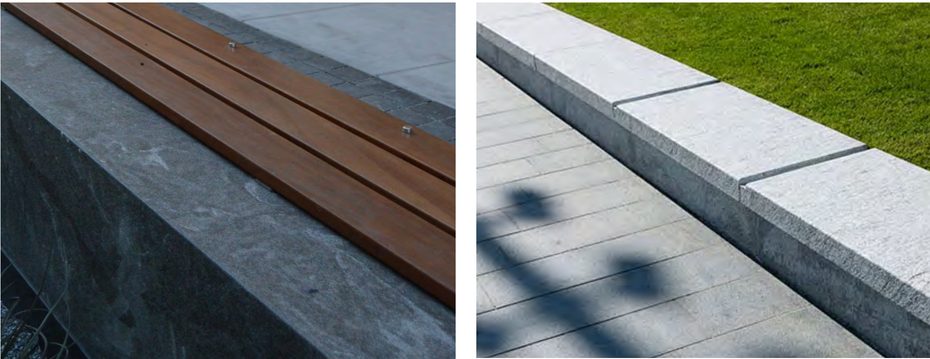
Cast-in-place concrete or precast concrete (to be determined) with wooden bench tops. Seating steps and seat-walls will be designed with anti-skateboarding elements.
