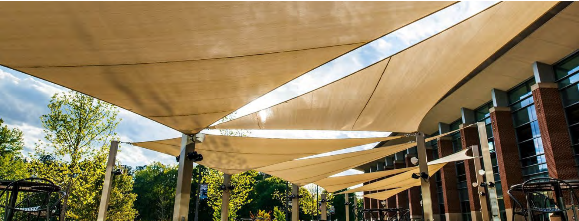
The proposed shade structure consists of tensile fabric shade panels with steel frame. (See renderings.) The shade structure would also support site and stage lighting and misters.
